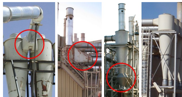
Figure 14. Cyclone design variations for the tested systems (left to right): dual configuration that splits flow between identical 1D3D cyclones with 2D2D inlets; 1D3D cyclone with an inverted 1D3D inlet; 1D3D cyclone with 2D2D inlet and expansion chamber on the cone; 1D3D cyclone with 2D2D inlet and standard cone.
